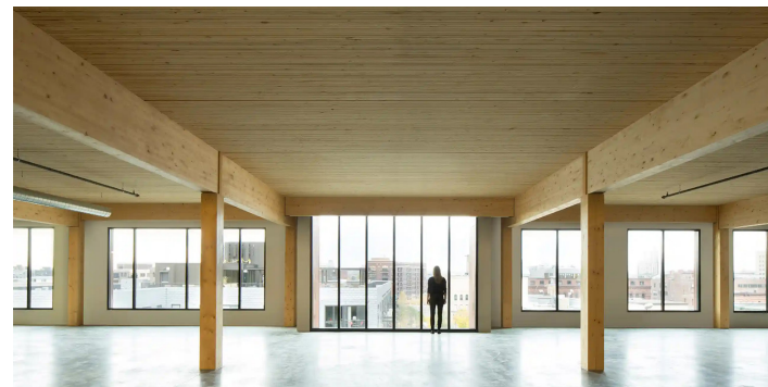
Mass timber building with expressed timber elements
